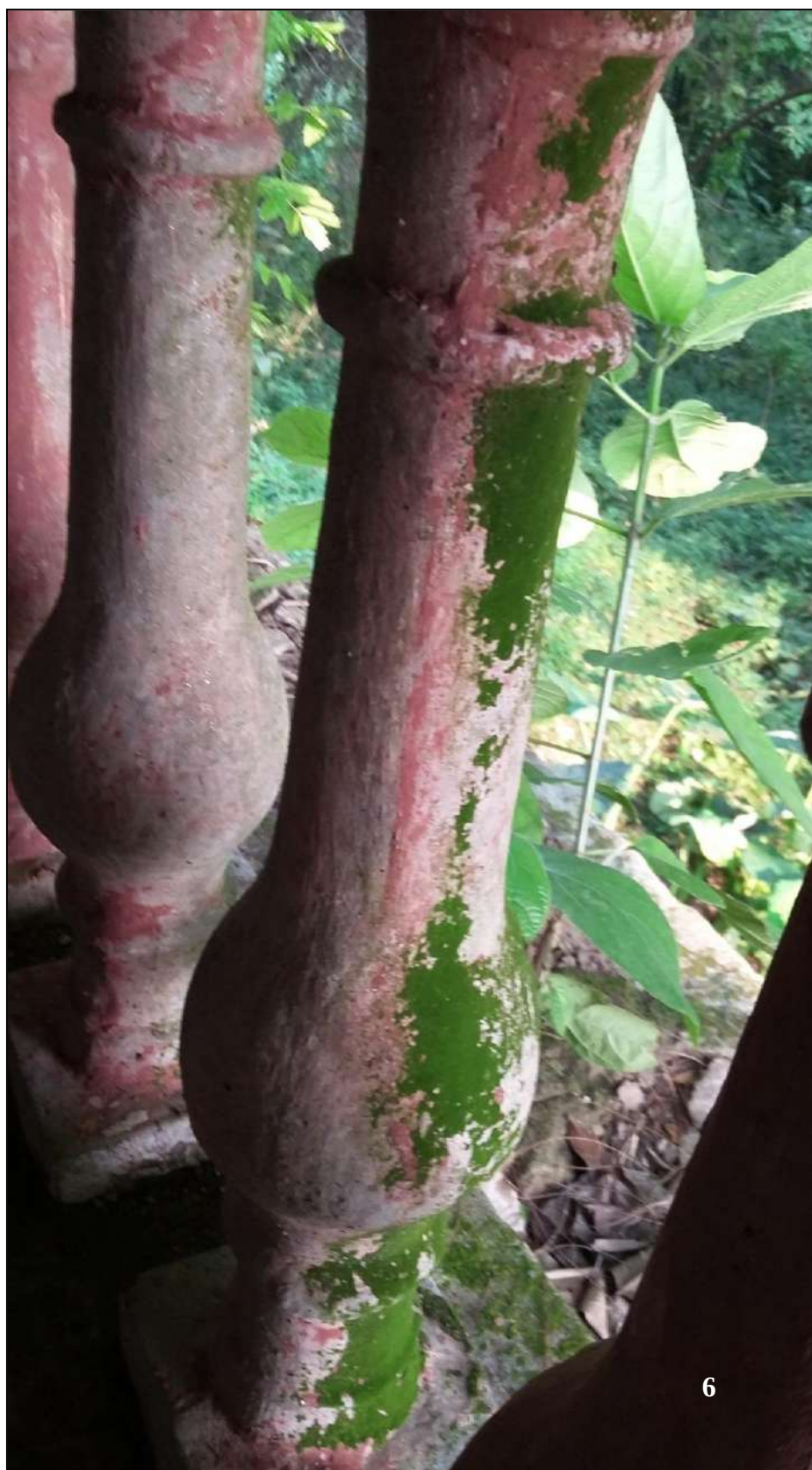
Photo 6. Close-up of green algal patches on Roxburgh Building
