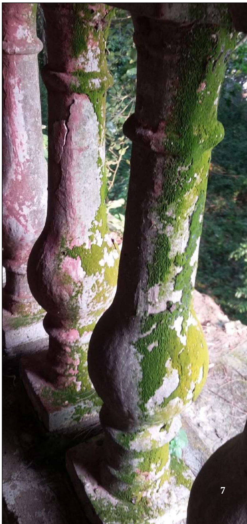
Photo 7. Close-up of greenish yellowish algal patches on Roxburgh Building
