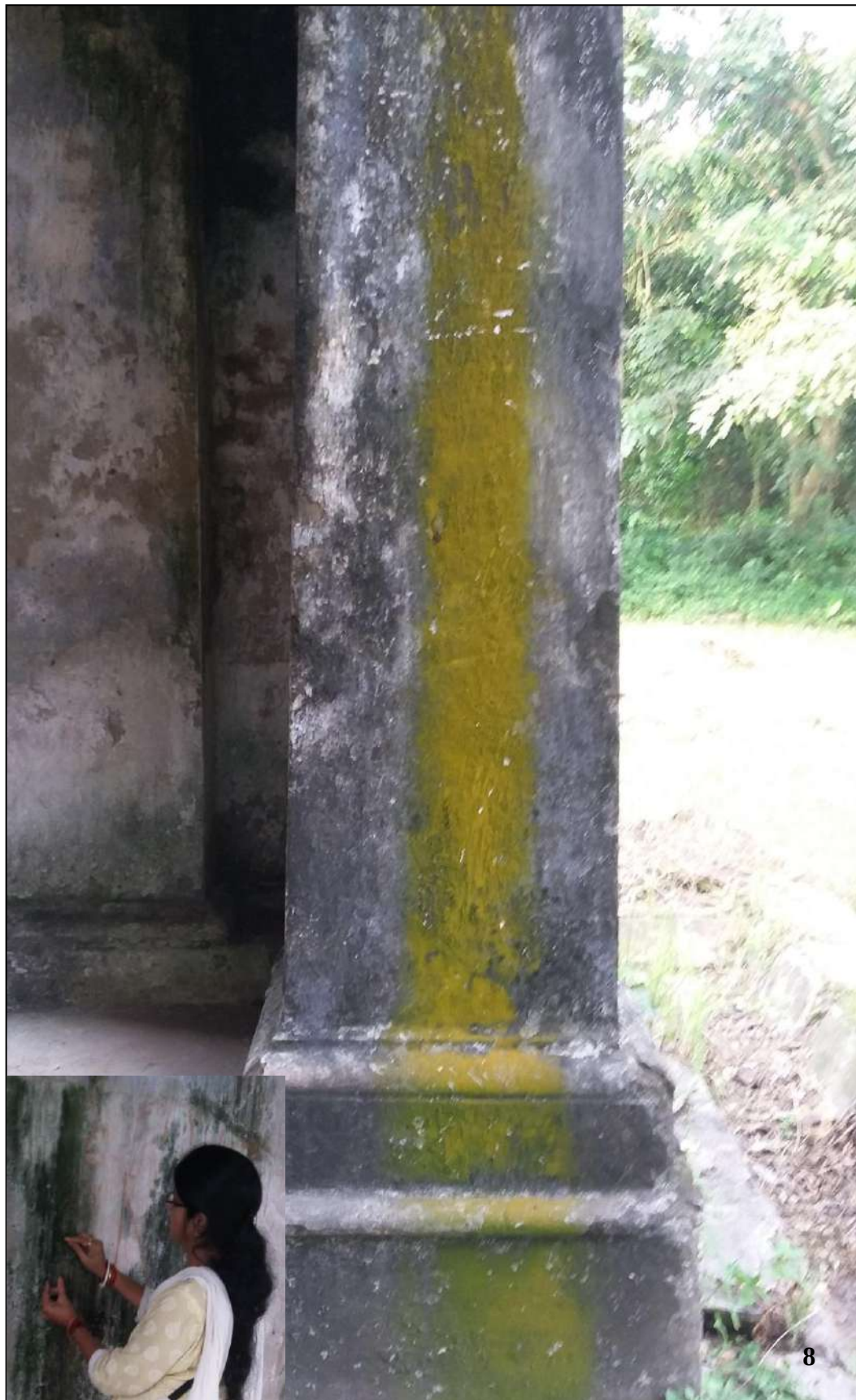
Photo 8. Close-up of algal patches on Roxburgh Building
