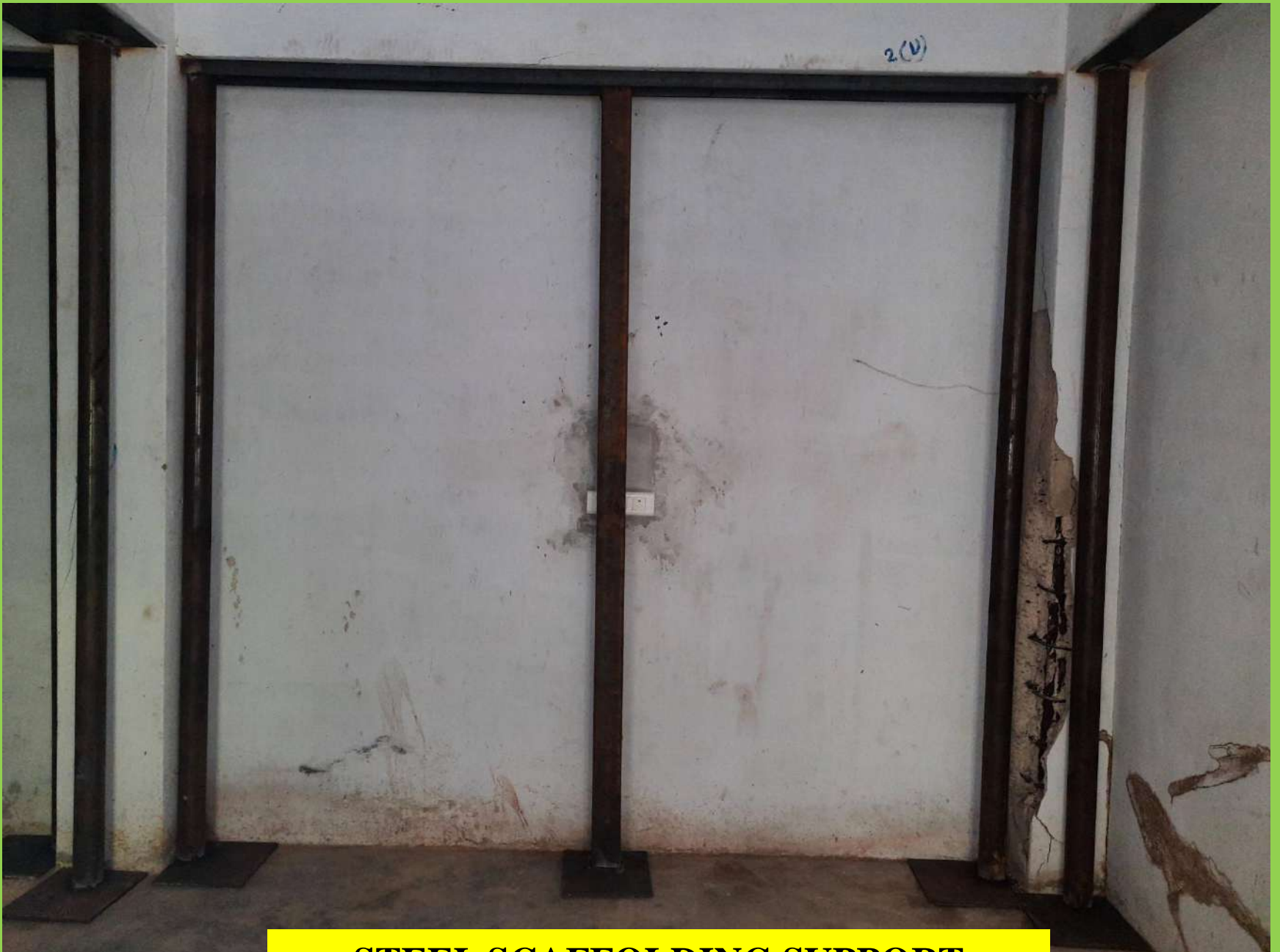
STEEL SCAFFOLDING SUPPORT
