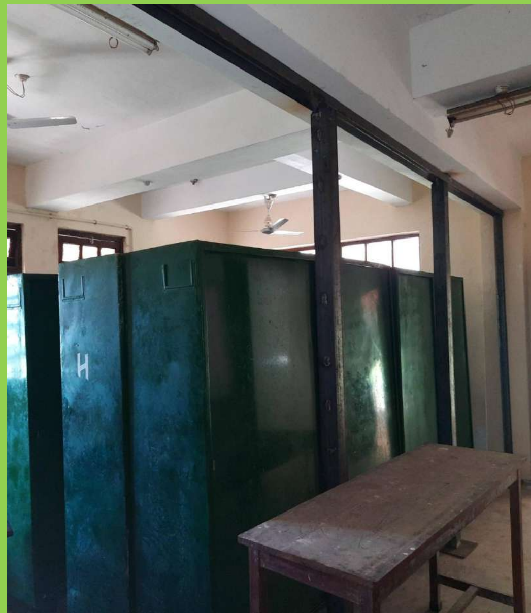
STEEL SCAFFOLDING SUPPORT
