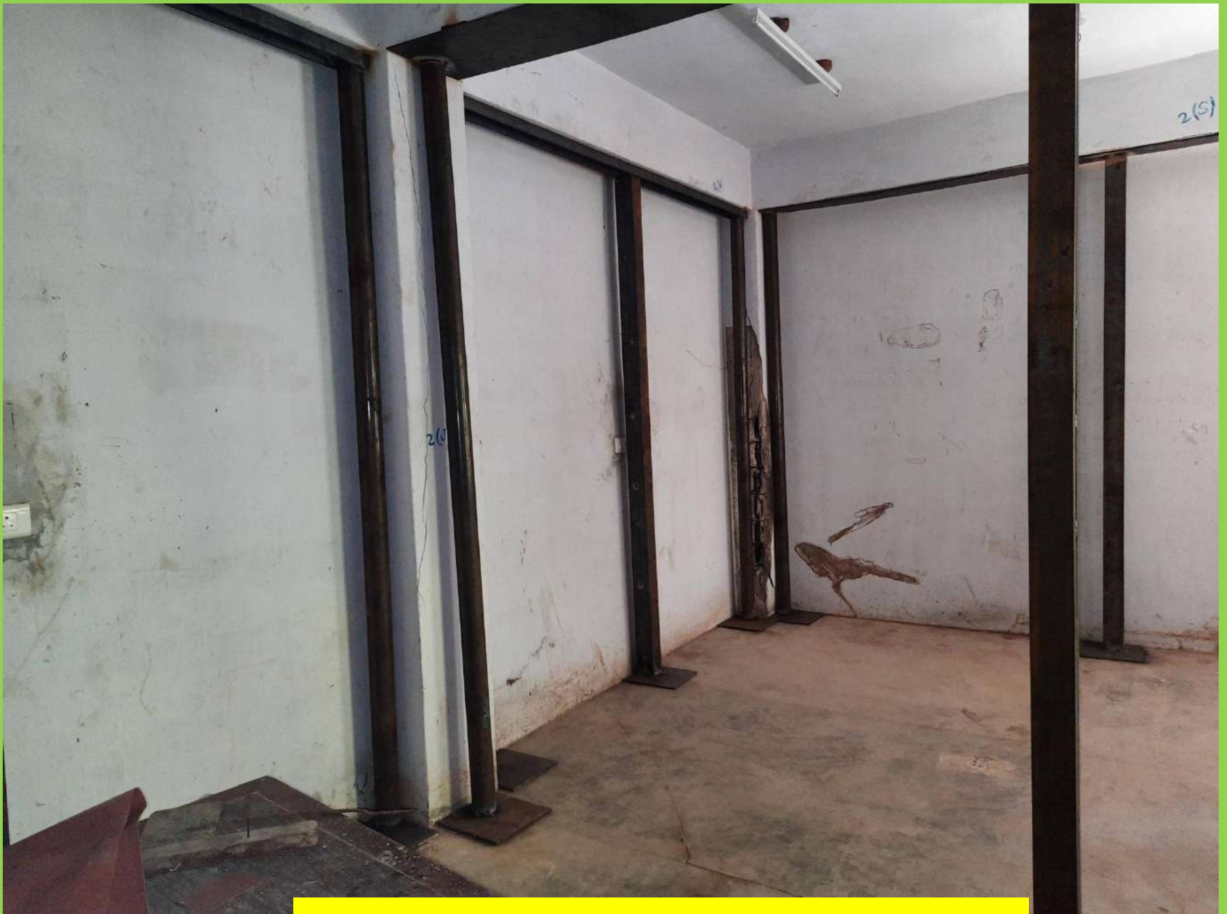
STEEL SCAFFOLDING SUPPORT
