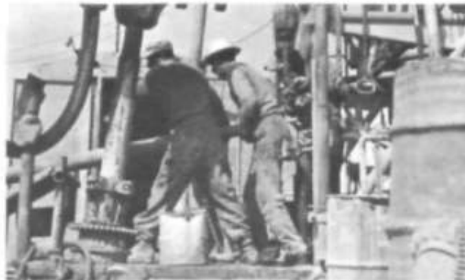
Another section at pipe goes if own in (ht wrch lot ontjat ground water in Jantwn % southern desert
